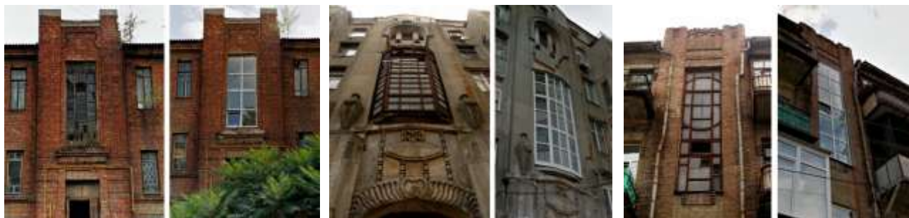
Fig. 4. Replacement of timber window sash structures with loss of the pattern of divisions (left to right): 30 Hromadyans'ka str., 20 Mykolaivska str., 14 Vorobiova St.
