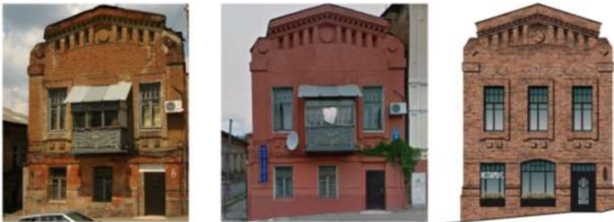
Fig. 14. Proposed facade reconstruction of “brick art nouveau” style building on 8 Bursatsky Descent, Kharkiv. 2008, 2015 photos & graphic reconstruction option of the façade
