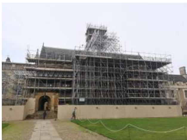
Fig 9. The Hall during restoration. (Photo by Volodymyr Meshcheriakov)
