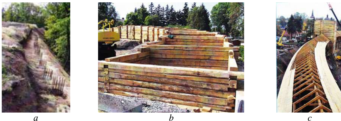
Fig. 6. Reconstruction of defensive walls and fortifications of the Baturyn citadel (2008): a – strengthening the slopes of the citadel; b – construction of load-bearing structures of defensive walls; c – installation of the tower and covering of defensive walls.
