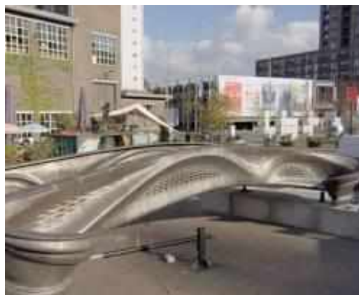
Fig. 15. 3D printed bridge with complex geometry
