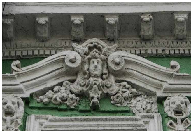
Fig. 10. Mercury on the facade of the house
